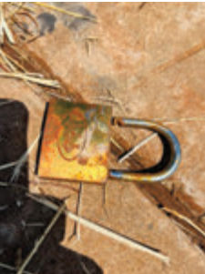
Locks and covers at the Y-piece were broken.
